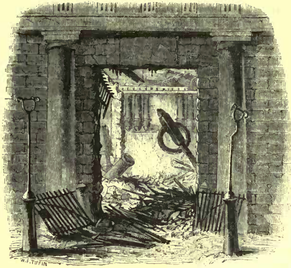
[Entrance, Staircase, &amp;c., of the Great Storehouse after the Fire.]
